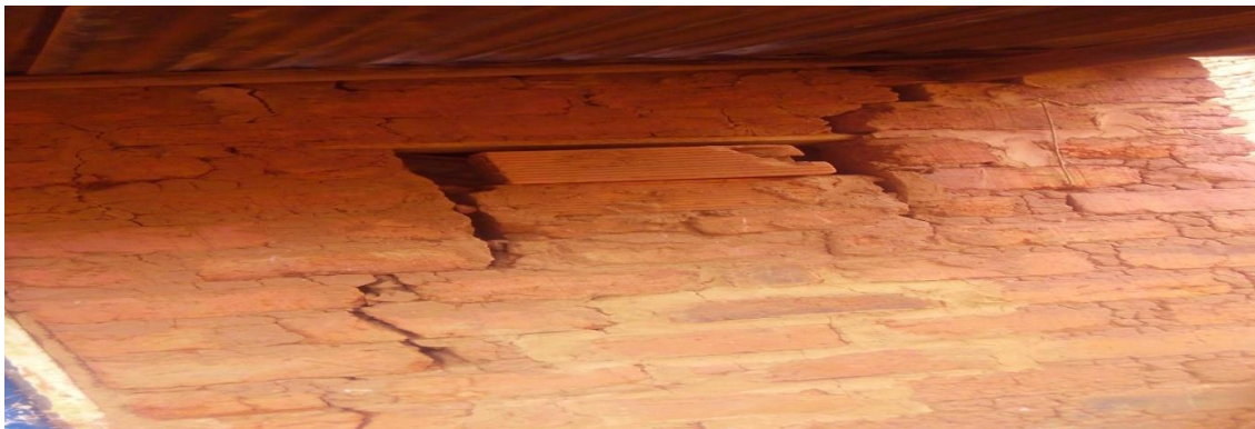
Cracks in the wall caused by rocks blasting in Kalukuluku
